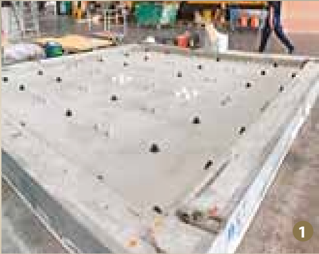
Arco DAMPING tracking and positioning.
