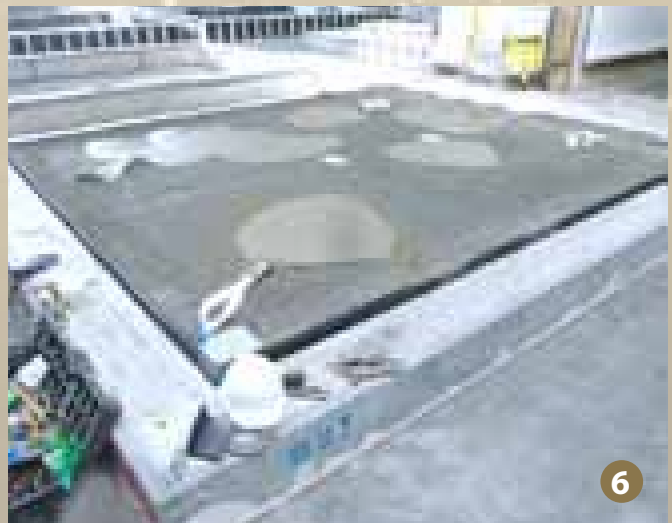
Arco MASS DAMPER leveling.
