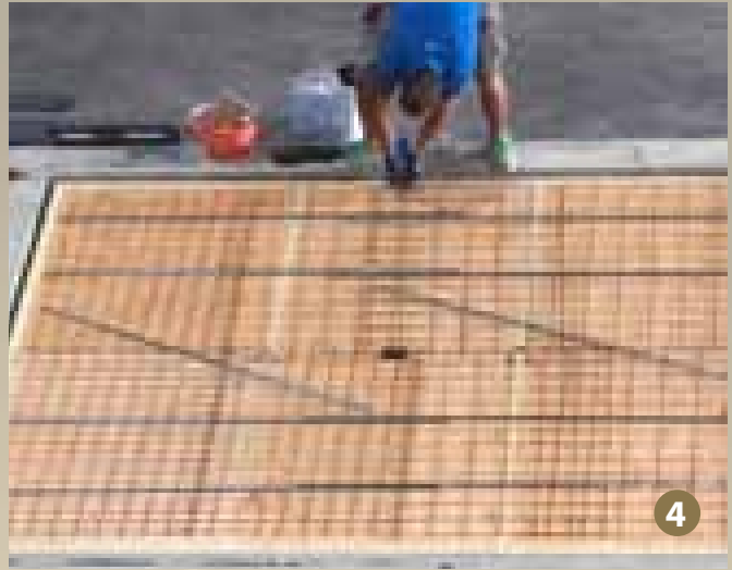
Welded mesh and steel bars application.
